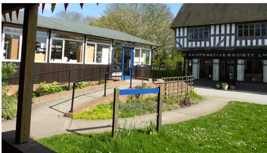
Ramped access from the Museum's shop
