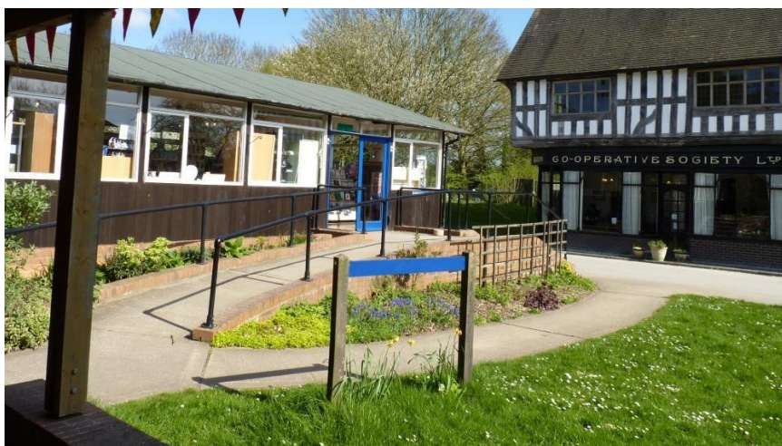
Ramped access from the Museum's shop
