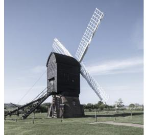
The windmill was near collapse in 1969 when it was carefully surveyed, dismantled and reassembled at Avoncroft Musuem. The windmill's move was completed in 1970. It took a further 7 years of careful restoration to get the windmill working,
