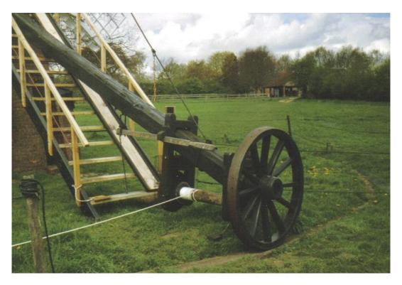
The white rope here is attached to a winch and is being used to help to turn the top of the wind mill so that the sails face into the wind.
